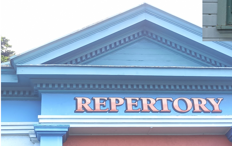
Figure 10: Close up picture of the existing central portal of the Repertory (once library) building showing the preserved mouldings and dentils. Note the lack of decoration within the triangle of the pediment that was typical of neoclassical detailing.
