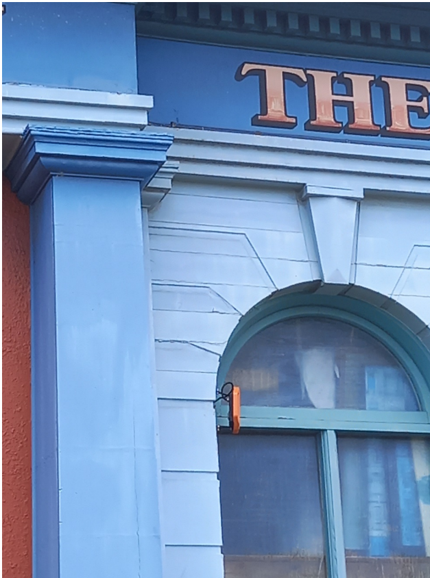
Figure 11: Existing Repertory Theatre façade showing the central 'keystone' detail over the front windows and the timber tongue & groove façade cladding cut to resemble stonework detailing. To the left is one of the reconstructed timber columns apparently installed during renovations in the late 1950's replacing the original curved ones.
