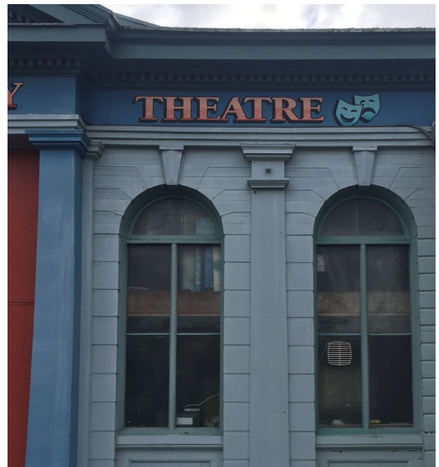
Figure 18: Front façade showing mezzanine floor built across window openings.
